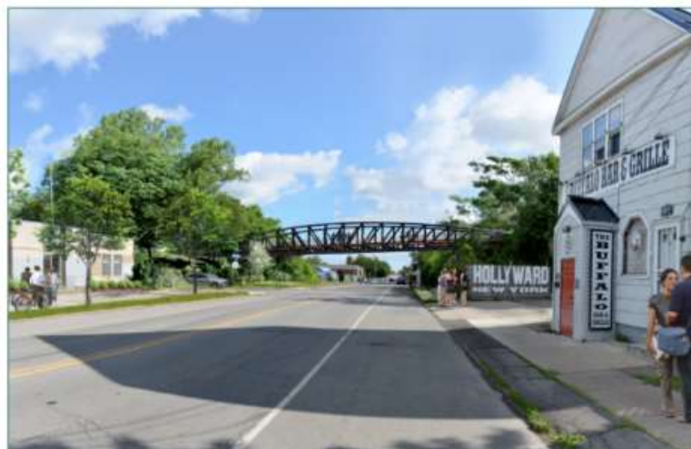
View north of Louisiana St. Bridge
