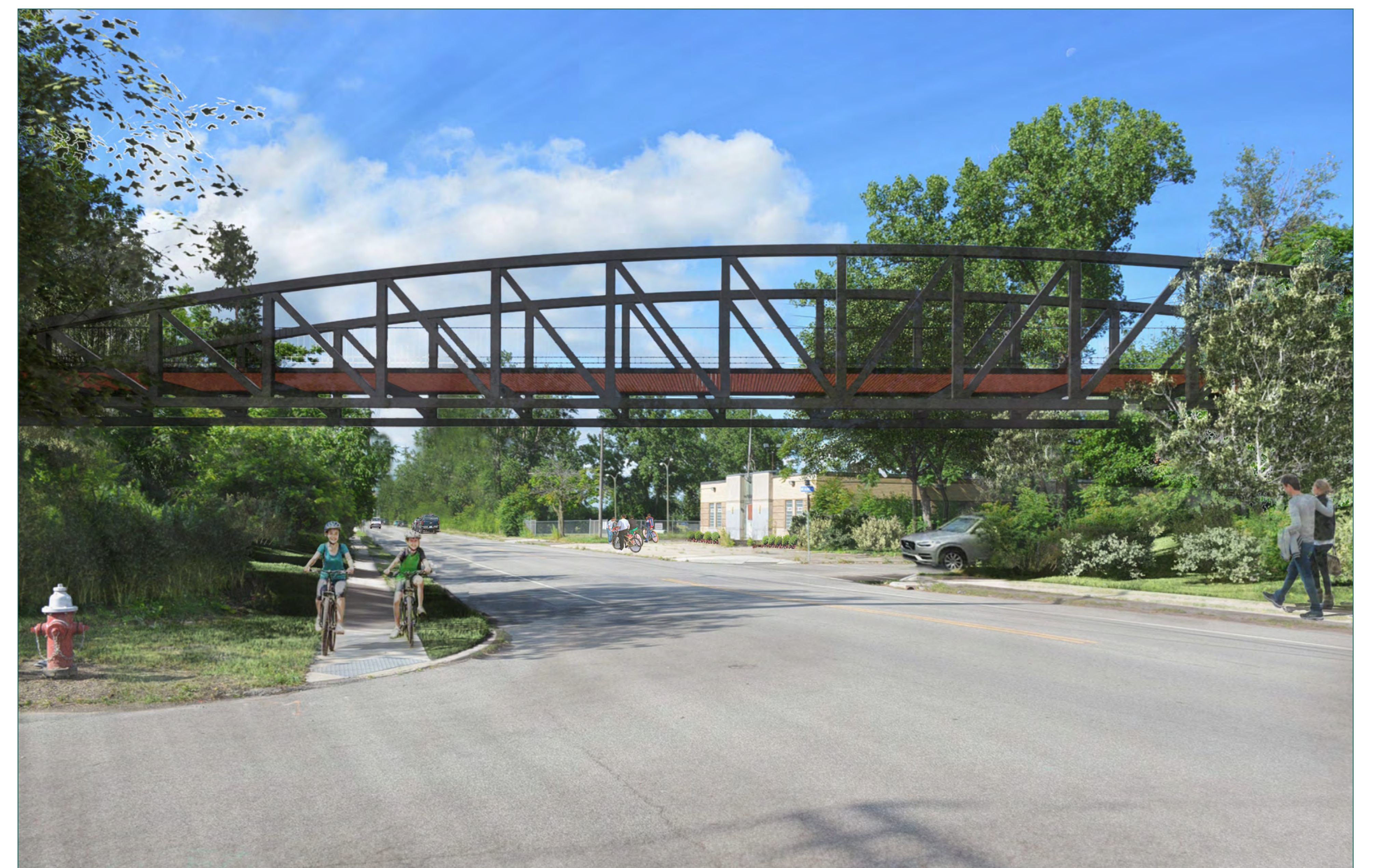
View south of the Louisiana Street Bridge
