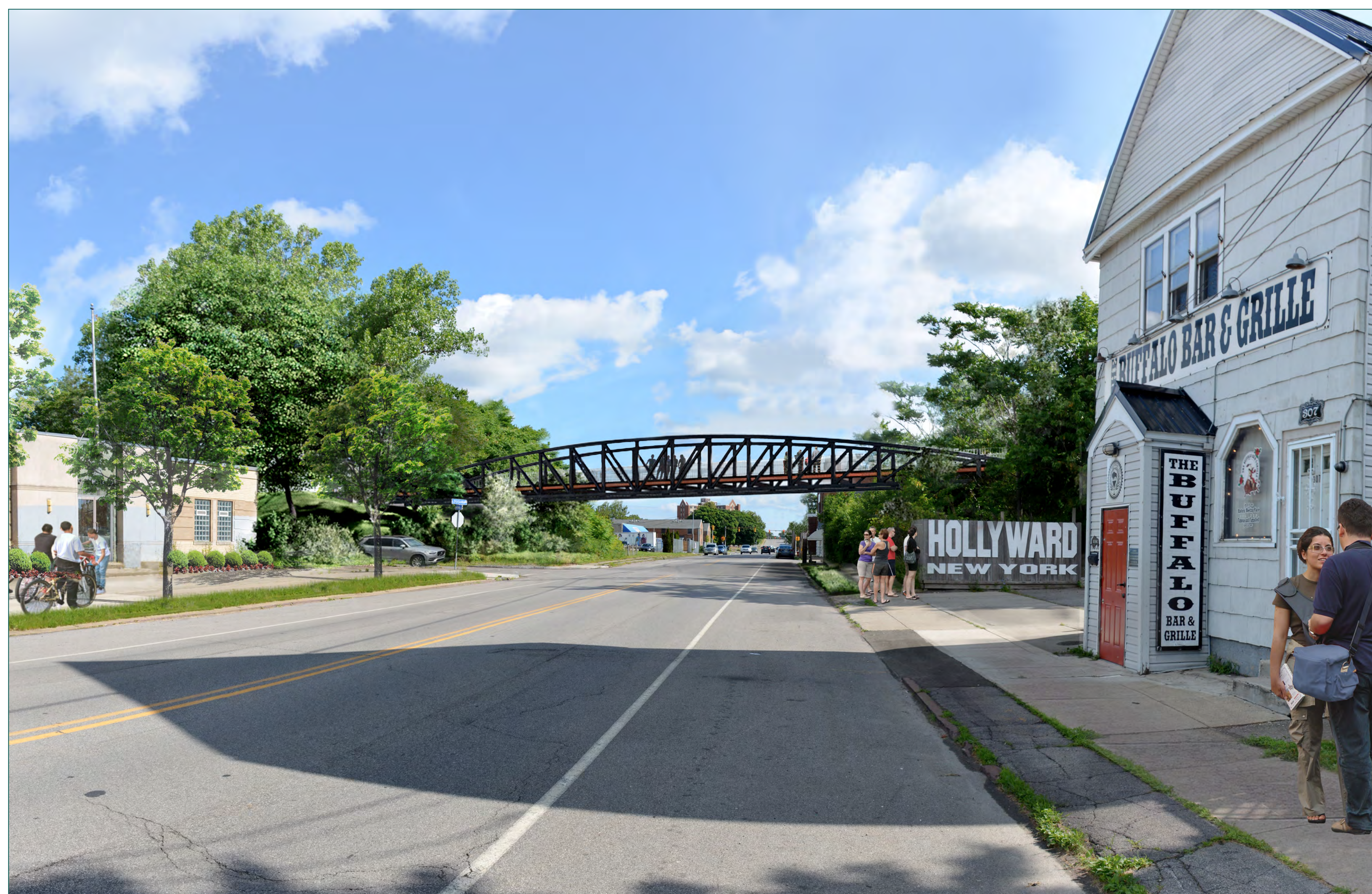
View north of the Louisiana Street Bridge
