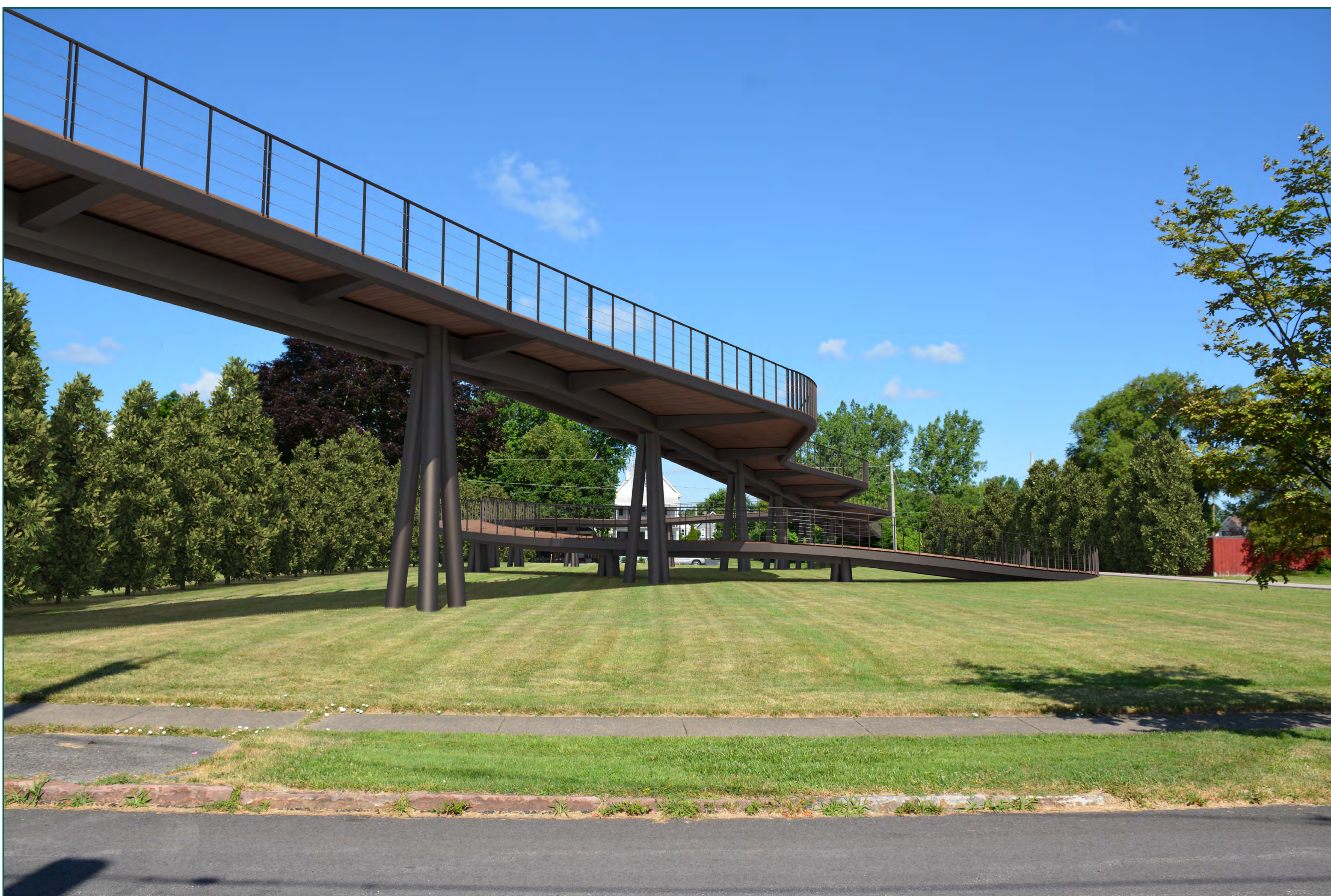
View west from Fitzgerald Street looking toward the Junctures Trestle Bridge
